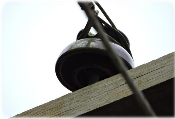
Pin Insulator Crack
